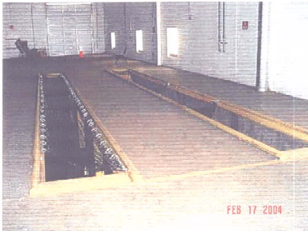
Photograph 1: Vehicle service area (subsurface) inside the warehouse on Parcel 1.
