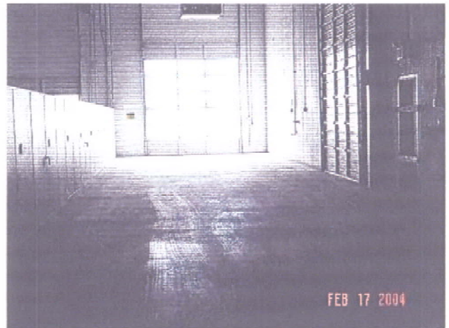
Photograph 4: Loading/unloading area of warehouse (northeast side).
